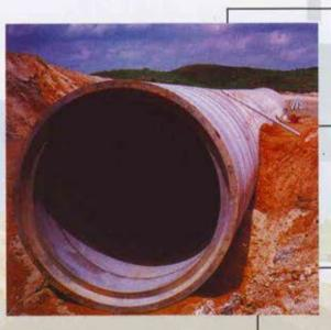
Test Load kN/m **Nominal Approximate** To MS 881 - 1991 **Nominal** Weight Length Diameter H per pipe M (M) (mm) (Tonne) Ultimate Proof Ultimate Proof Ultimate Proof Load Load Load Load Load Load 230 2.50 7.04 146 183 184 120 96 2.50 8.75 108 135 165 207 210 263 2.00 8.51 294 124 155 186 233 235
